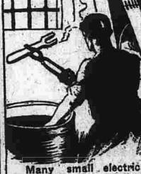
Many small electric furnaces are used in industry for making tools. Tools are hardened in salt baths liquefied by the electric arc.
